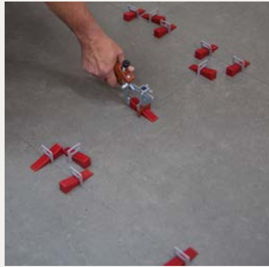
For large format as 30x90, 60x60 and 60x120 cm the use of leveling systems between parts is compulsory for perfect installation (picture wedge levelling system).
